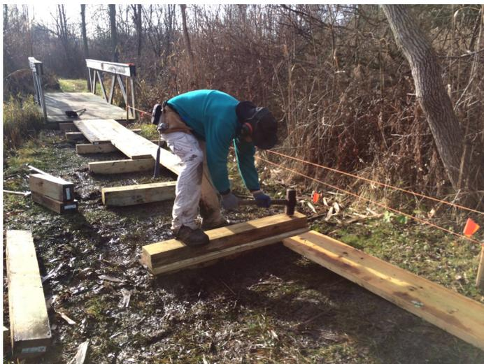
Chauncy driving re-rod into the ground.
