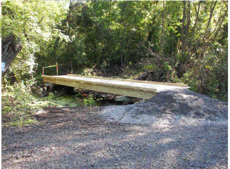
The bridge shown here is nearly complete. Stone approach ramps on both ends have been put in place.
