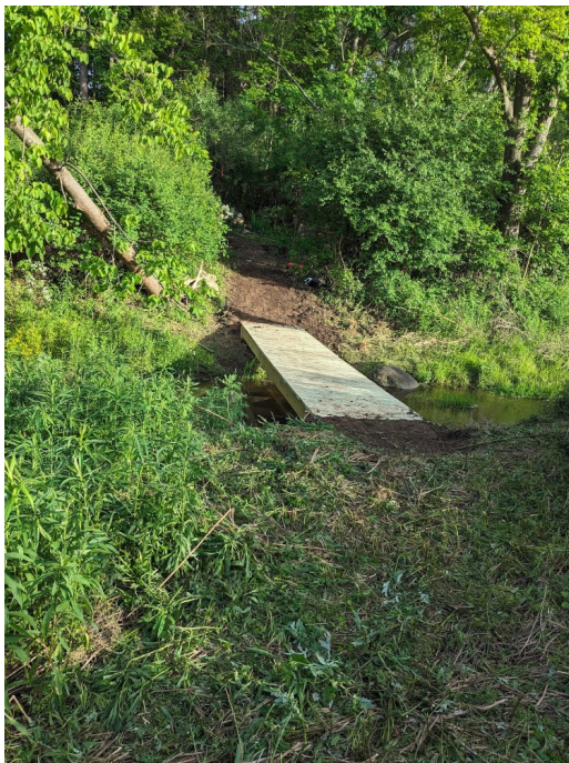
New temporary bridge.
