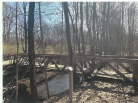
Domine to Auburn bridge
